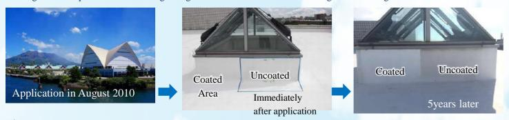
◆ Tokyo Big sight West building's roof / Anti-fouling coat on thermal barrier painting
