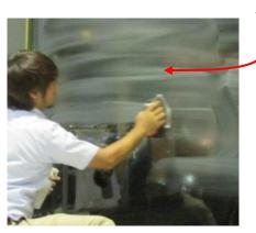
When there are many parts of oil film, it is better to use the polisher machine to polish the glass.
