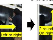
⑤When you come to the right sash frame, apply the sash frame vertically for at least 2 round trips.
