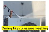
"Be cautious during high-pressure washing of the outdoor unit, as there is a risk of water getting into the circuitry and causing damage."
