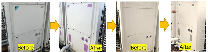
"When covering the outdoor unit, there's a possibility that it may get buried under the paint, making it difficult to identify during removal. Try to avoid painting over it, or if you paint over it, do so in a way that the seal marks are visible. In the worst case where it's unclear, take photos in advance to confirm the areas that were covered before removal."
